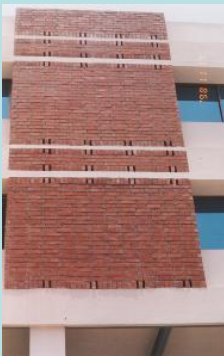
CONSTRUCTION OF CAVITY WALL
