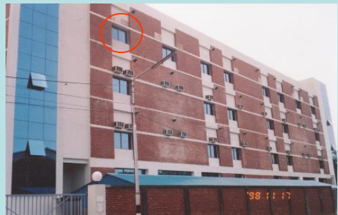
RECESSED WINDOW FILLED WITH TINTED GLASS
